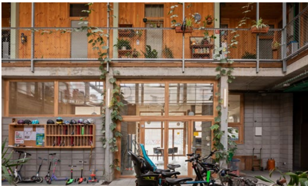
La Borda , Barcelona is a self-organised housing cooperative offering sustainable, non-speculative housing. The project is located on a public land of social housing, with a leasehold of 75 years. Here you can see its collective living spaces and timber framing, built by its own timber framing construction cooperative. Photo: Ivaro Valdecanto.
