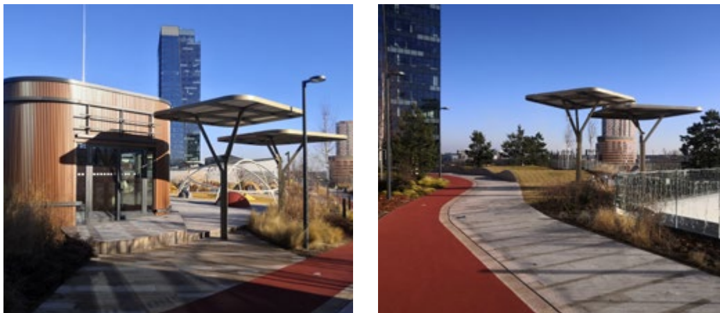
Figure 1: Green roof of the NIVY Shopping Centre with a view of the NIVY TOWER in winter 2024 with a playground and a jogging path in the background. Source: own pictures.
